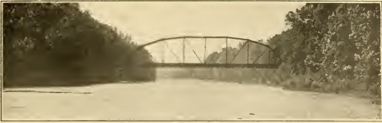
Chesapeake-Western Bridge across the Shenandoah River near Elkton
